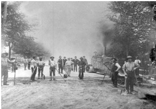
Workers on Jarvis Street
